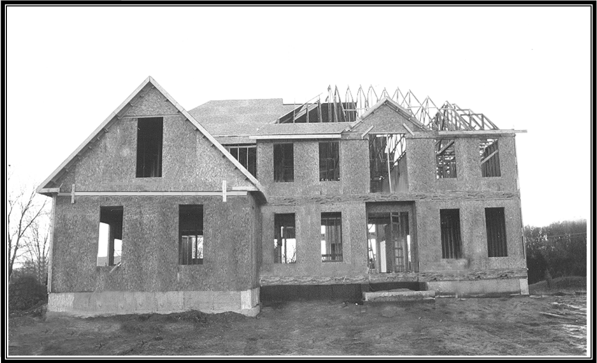
FIGURE 1.2 Modern Platform-Framed House under Construction
