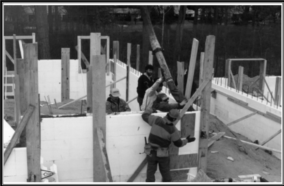
FIGURE 1.5 House Construction Using Insulating Concrete Forms
