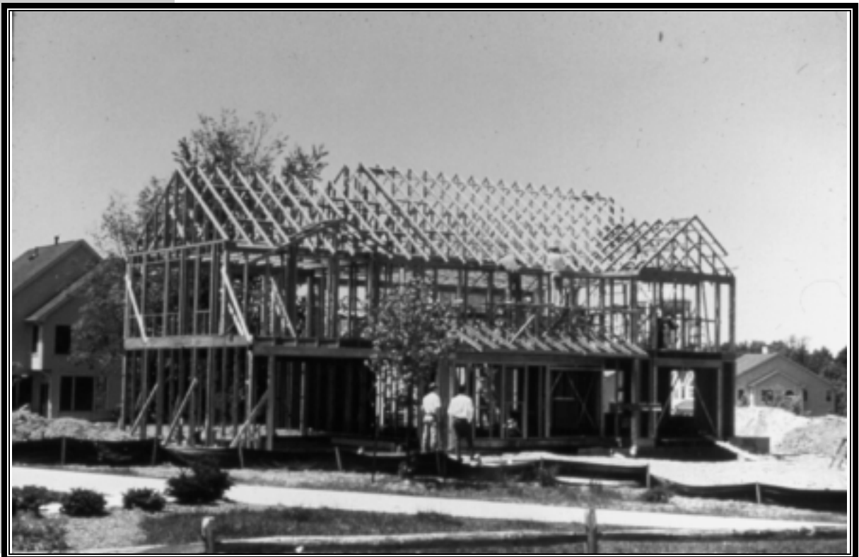
FIGURE 1.4 House Construction Using Cold-Formed Steel Framing
