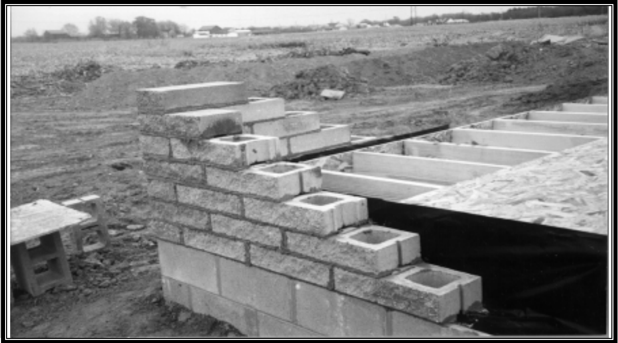
House Construction Using Concrete Masonry
