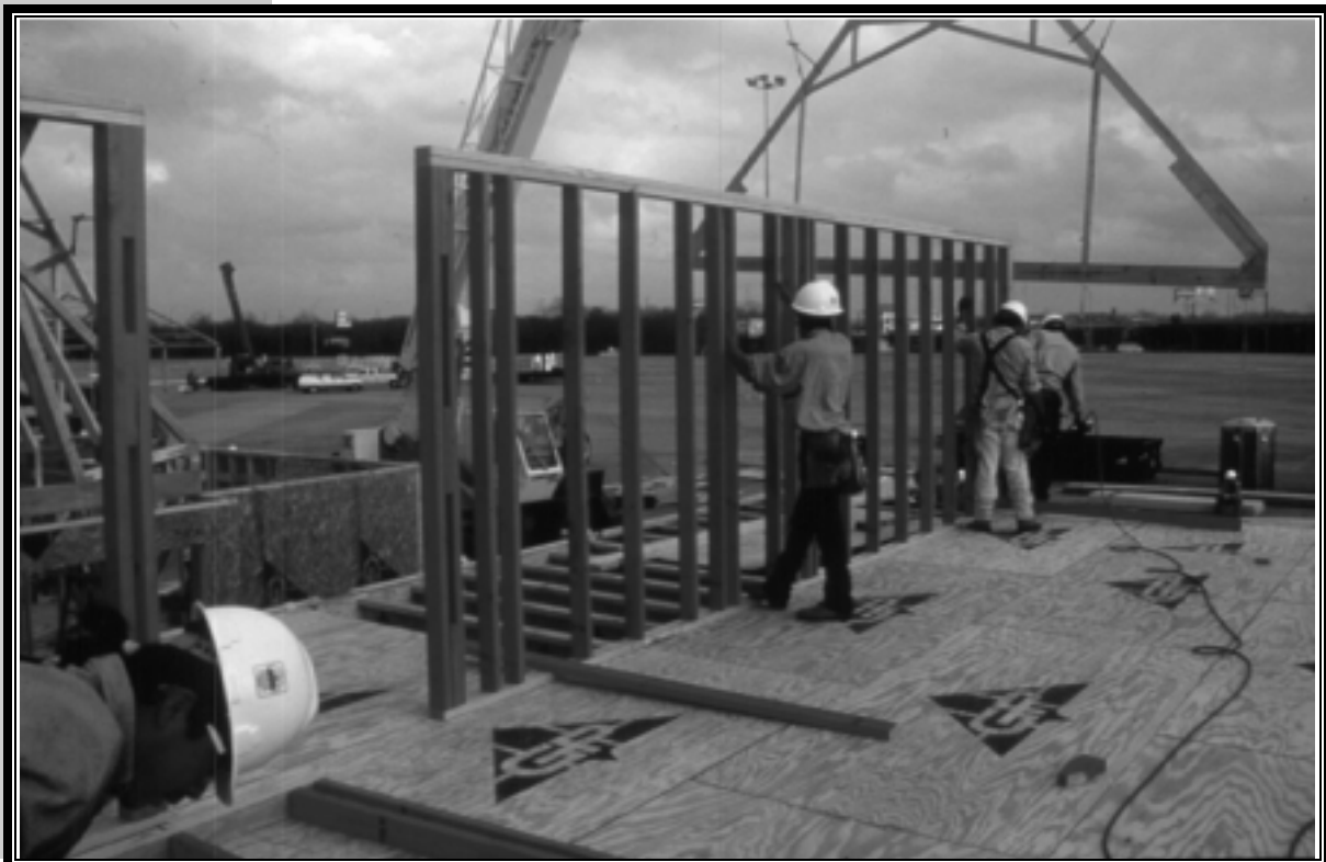
FIGURE 1.3 House Construction Using Engineered Wood Components
